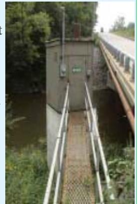
The picture below is one of the real time gaging stations on the Maumee River just east of Landin Road near New Haven, IN. This station has a radio antenna (shown to the right of the well), which enables communication. Additionally, please note the light colored line about half-way up the well which indicates that water spends some time on the well in that location (about 10’ higher than when this picture was taken.)
