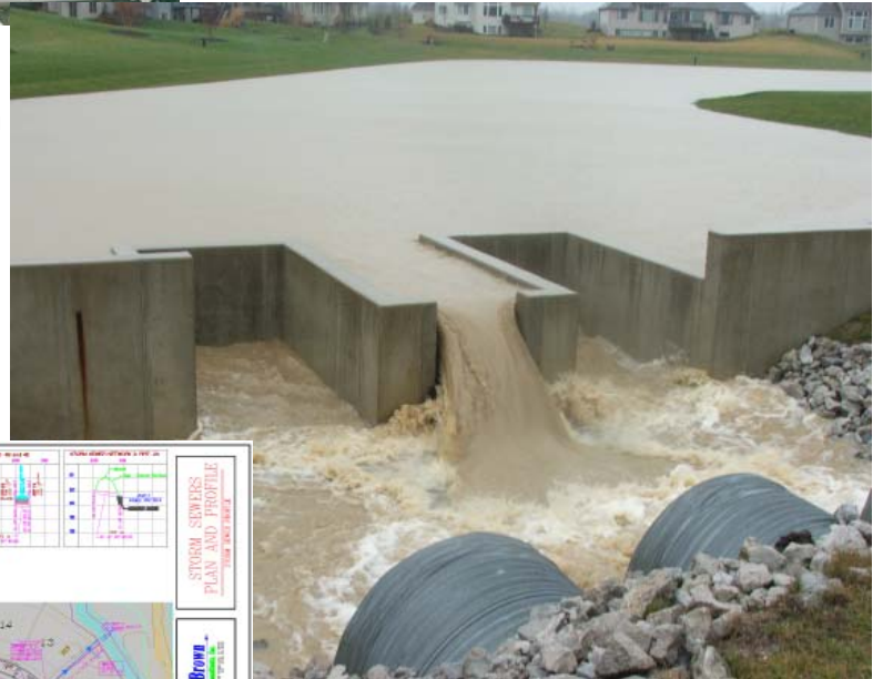
The Second Cascading Weir during a flooding event
