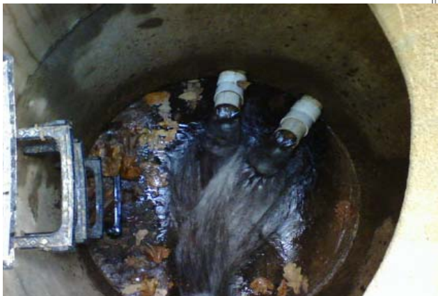
Photograph of one of the pond's discharge structure
