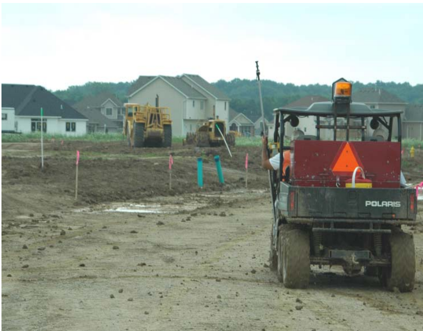
Typical construction staking site with Ranger ATV
